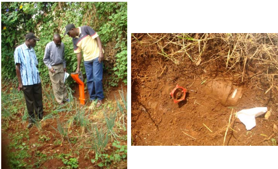
Plate 8: Unearthing a buried meter during pipe and metal locator demonstrations
